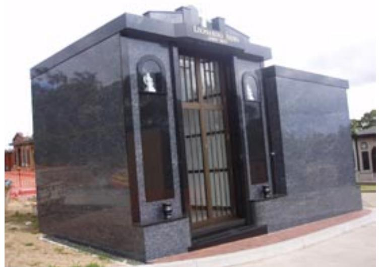
The use of aluminium in the doors of the crypts allowed a greater variation in their design. Lamination technology allowed glass to be used in the doors whilst meeting safety
