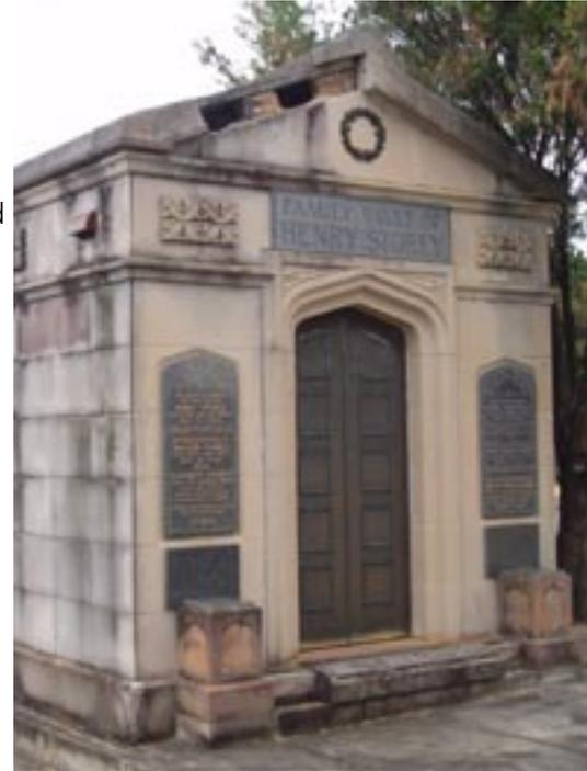
You may note the extreme weathering of the Storey crypt shown, especially the top left area of the roof.
